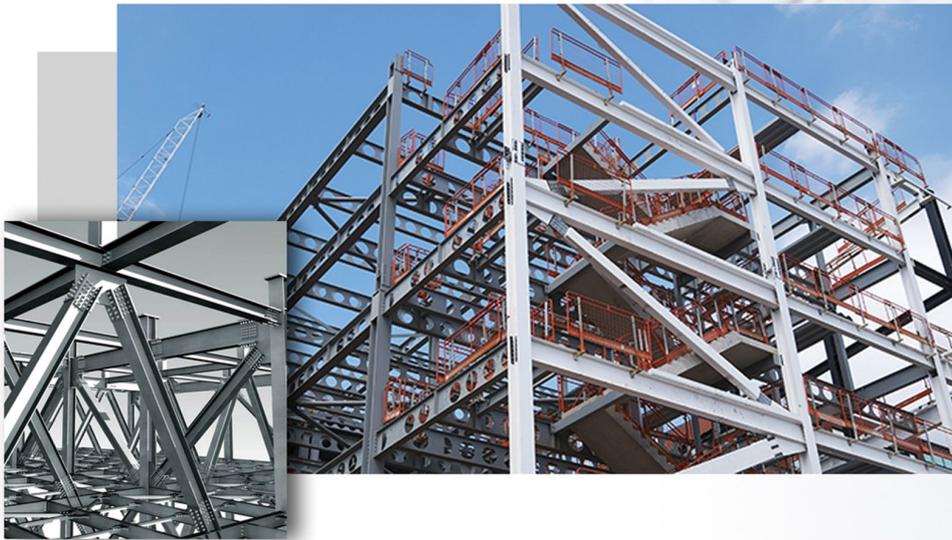
Building a high rise or any multi storey building demands the use of light weight yet strong materials. Steel, by virtue of its high strength to weight ratio, enables large span to light weight construction.
